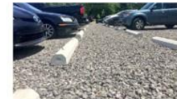
GRAVEL PARKING LOT
